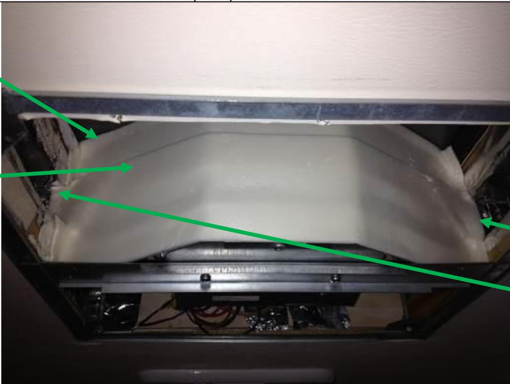
Extra insulation sealed against sides and fit into duct opening
