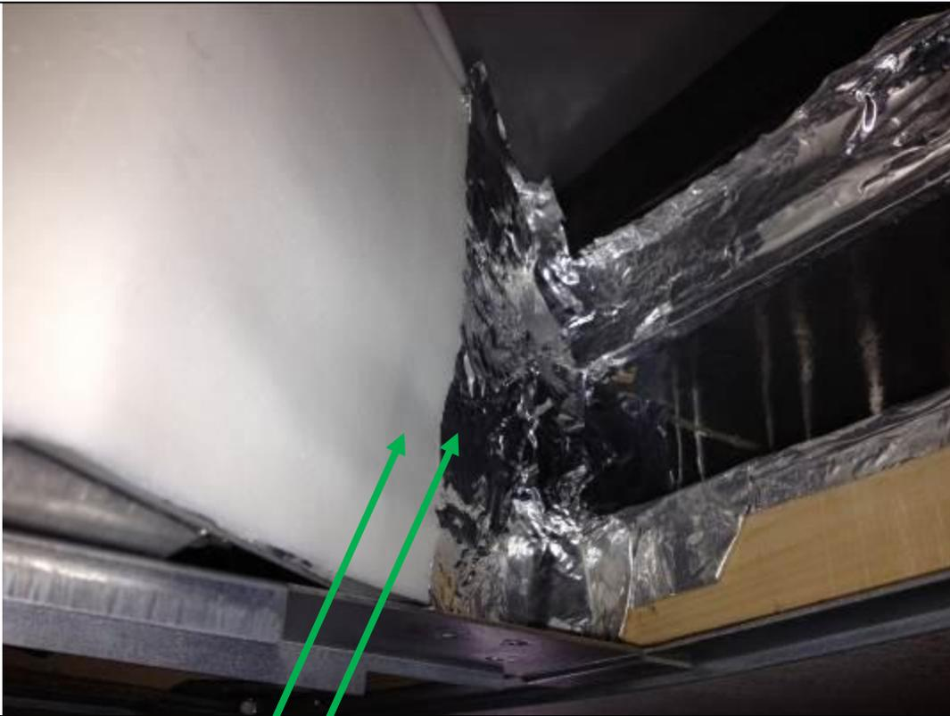
Additional tape to ensure duct is not restricted at supply opening and preventing recirculation at end of divider/insulation seal.
