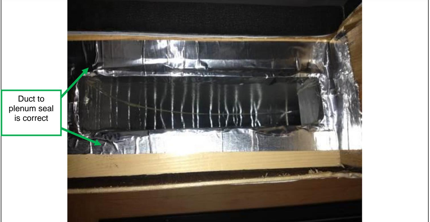
Correct sealing of supply ducts to supply plenum will provide maximum efficiency to duct system.
