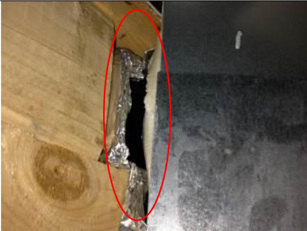
Divider not sealing supply and return air, which will cause recirculation and freeze (icing) condition and poor performance.
