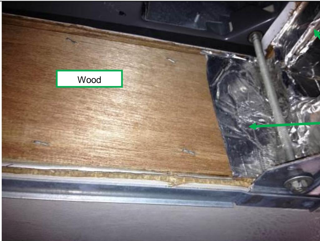
Proper AC opening preparation is important. Opening should be  $14 \frac{1}{4} \times 14 \frac{1}{4} \pm 1/8^{\text{th}}$ , refer to installation and operating instructions.
